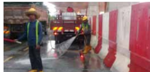
Truck wheels cleaning from soil
