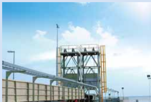
LEFT: Coal conveyor system at Tanjung Bin Power Plant, Johor, Malaysia
