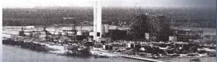
TRONOH CONSOLIDATED BHD - RECENT LARGE CONTRACTS
